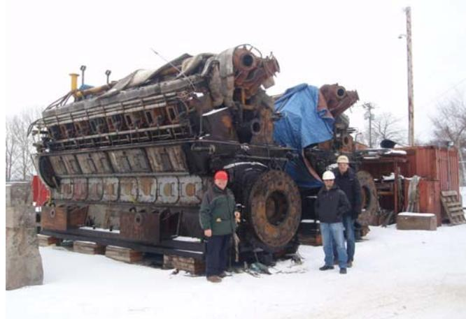
Preparing the space for the new engines took another couple weeks and then on the coldest day in December the new engines that weigh 117 tons each were set onto the beds in about four hours. When the crane operator brought the engines close to the mounting bolts the alignment was only a few millimeters off and the rigging crew could ease the massive machines into place.
