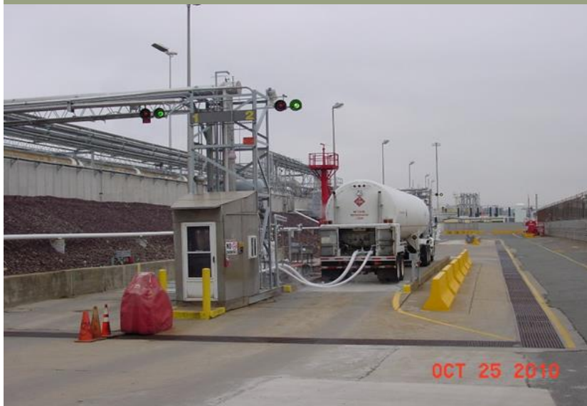
4 Trailer Loading bay at Distrigas' Everett terminal
