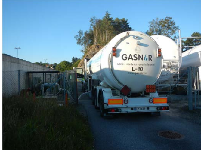
Resupply of LNG storage tanks from a road truck
