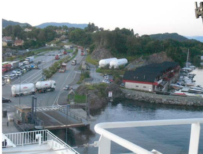
Dedicated 500 m 3 LNG storage tanks at ferry terminal in Halhjem, Norway
